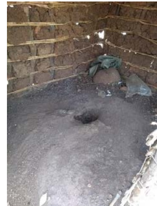
Figure 25 - A dirt slab latrine.
