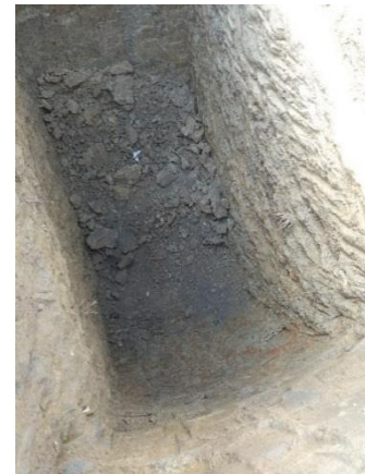
Figure 45 - A new, unlined shallow pit is under construction
