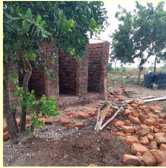
Figure 26 – New nursery school latrines currently under construction.
